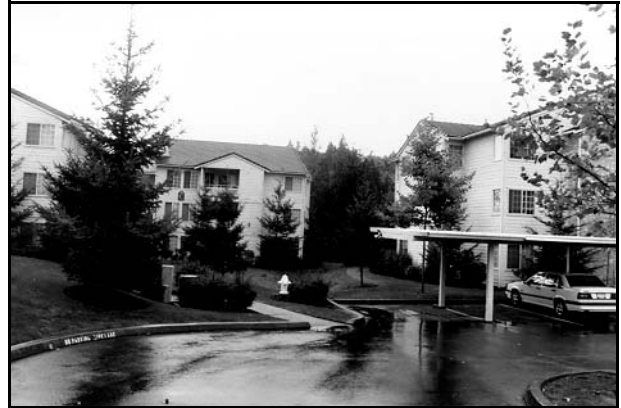
The Park at Forbes Creek Apartments
